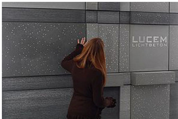
Fig. 2.13 View of translucent concrete wall at Expo Bau 2011, München/Germany
